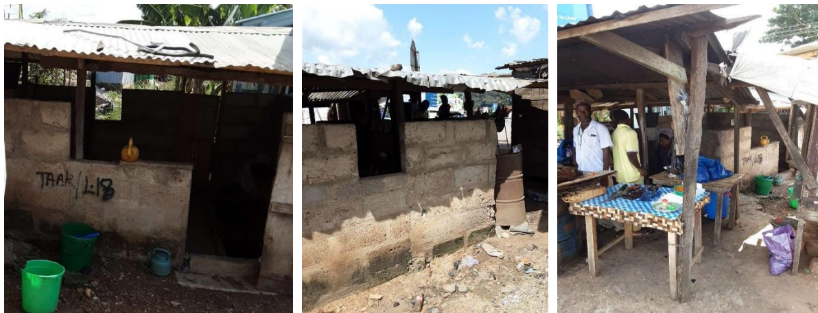
Figure 7-10 Religious Building and Attached Shed
